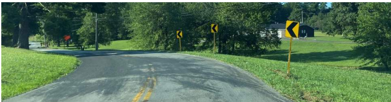
PHOTO 2: SB APPROACH NEAR ALSIP TRAIL
