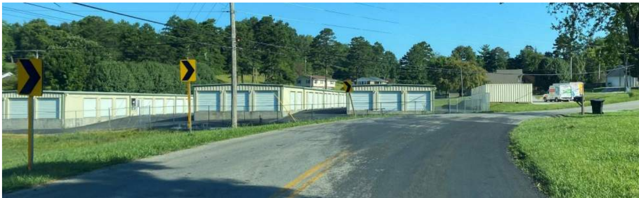
PHOTO 1: NB APPROACH NEAR ALSIP TRAIL
