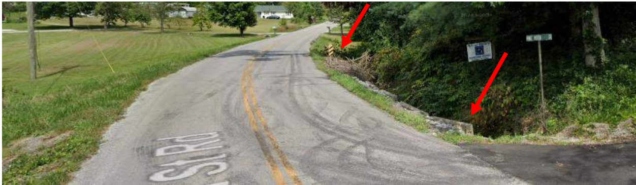
PHOTO 3: 5 TH STREET ROAD (EB) AT PINEWOOD DRIVE
