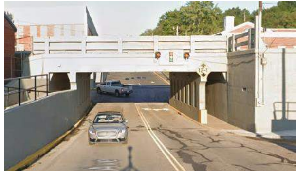
PHOTO 2: EB ROY KIDD AVE APPROACHING DEPOT ST
