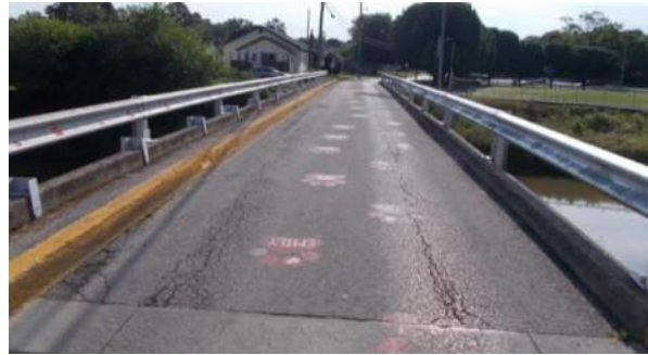
PHOTO 2: FRANK SELVY WAY AT BARBOURVILLE (NB)
