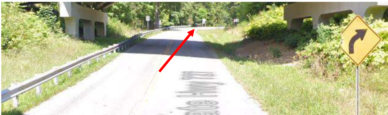
PHOTO 5: 5 TH STREET ROAD (EB) AT SCUFFLETOWN RD
